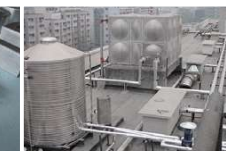
Water tank fabrication
