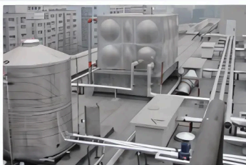
Water tank fabrication
